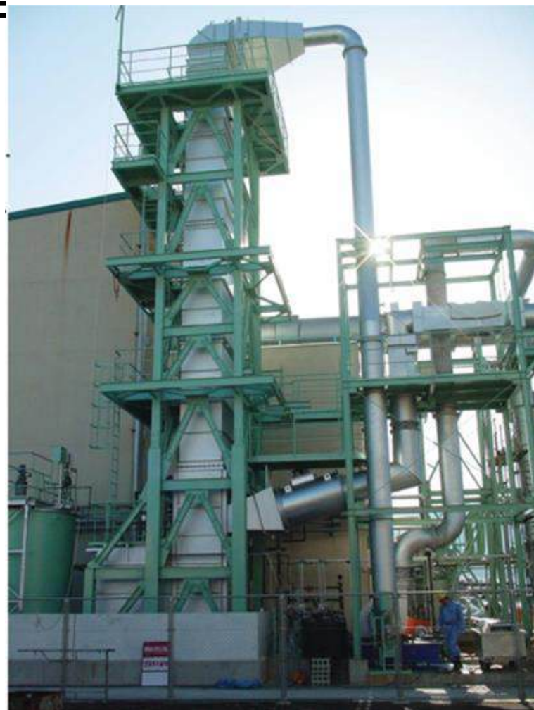
PDU for SOx Removal by ACF
